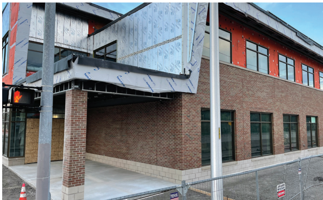
The Detroit Food Commons, under construction.
